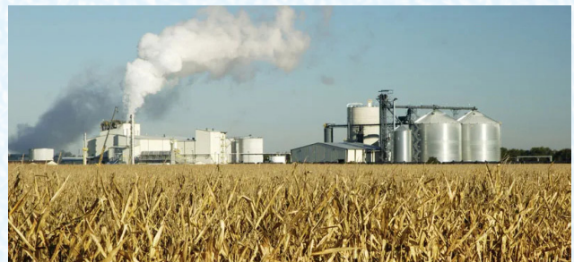
Fig: 2G Biofuel (ethanol) Production Plant
